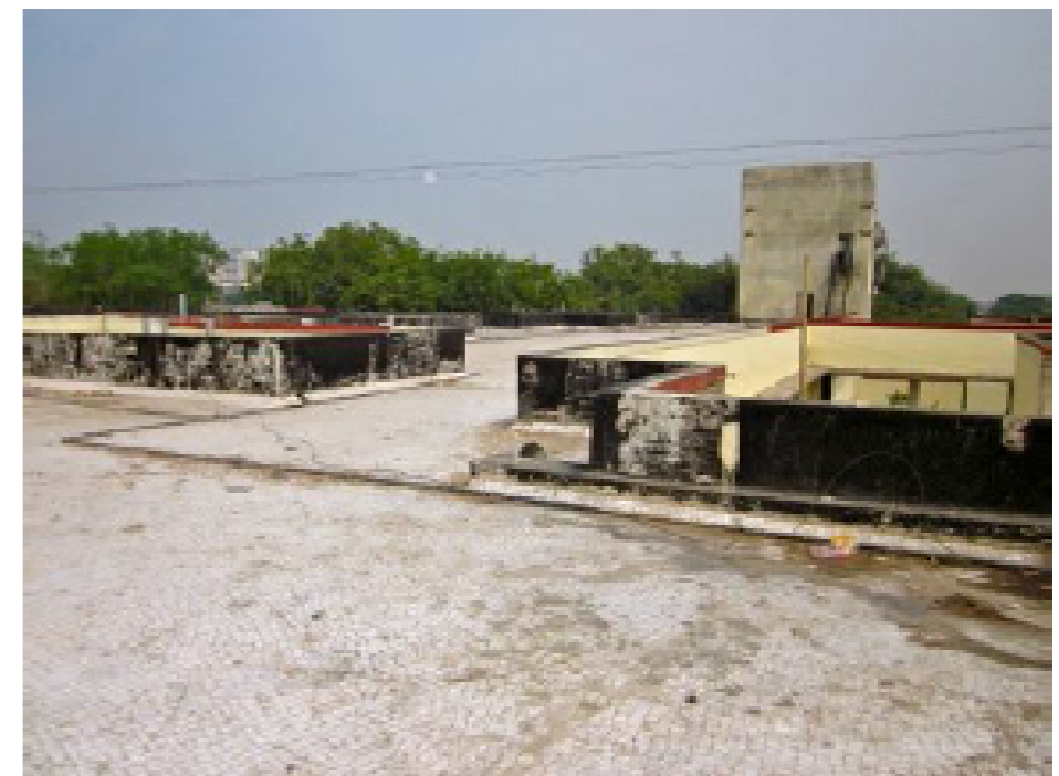
Roof replacement with china mosaic
