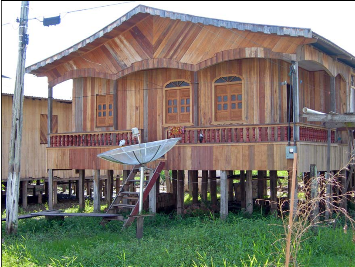
Figure 2 – A typical stilt wooden house in Anamã, with its own television antenna (Photo by Rita Pestana, July of 2006).
