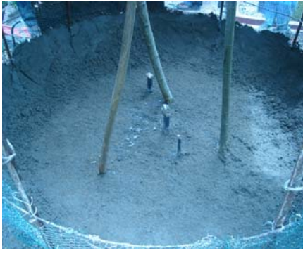
Various stages of the building process of an On-Surface/Above-Surface RWH Unit at Idamelanda, Left – concreted base and wire mesh reinforcement, Middle and Right: Application of mortar to roof. Photo Credits: Janaki Chandimala, 2008.
